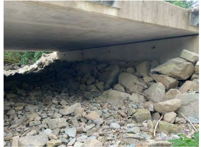
Left Bank Abutment when facing downstream
