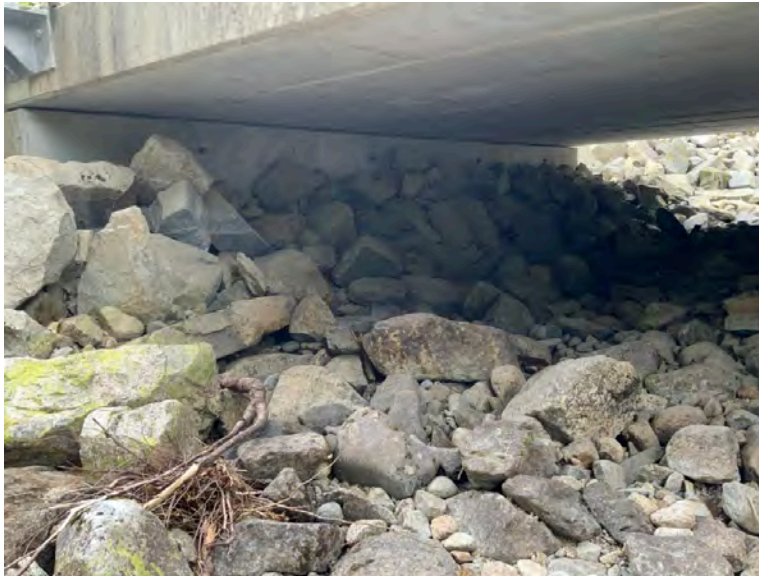
Right Bank Abutment when facing downstream
